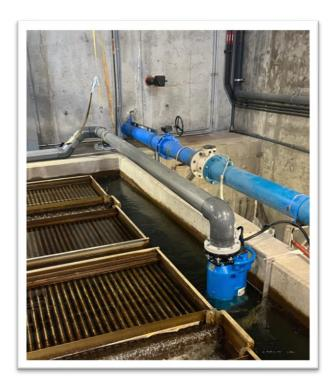
A new, temporary pump has been installed in the sedimentation basin at Signal Hill.
