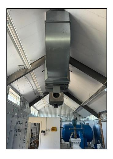
Completed Insulation Repairs at Old Ranch Road Booster Pump Station
