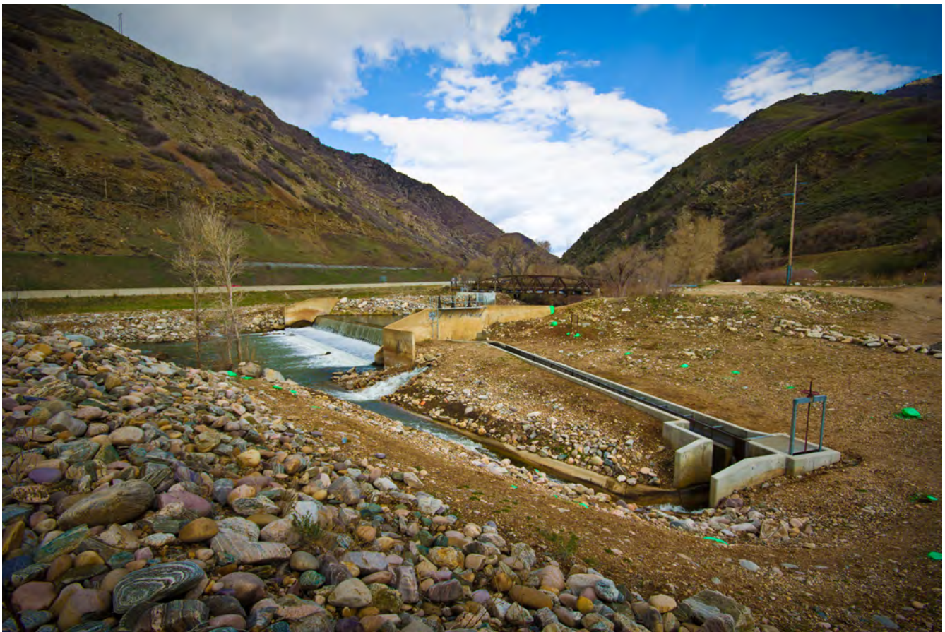
Fig 5.4: Fish Passage and screening structure at Weber Canyon
