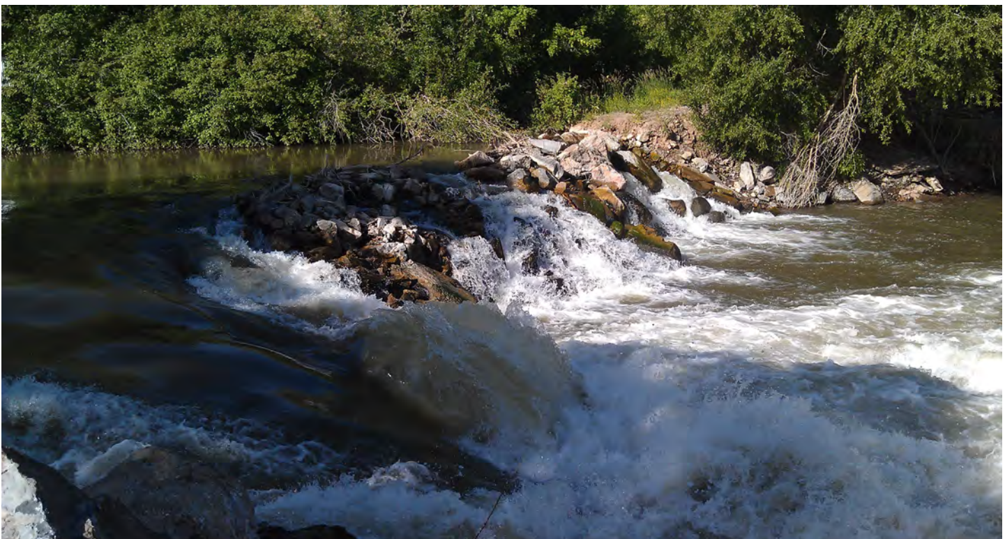
Fig 2.8: One of many low-head irrigation diversion dams in the Weber River watershed.
