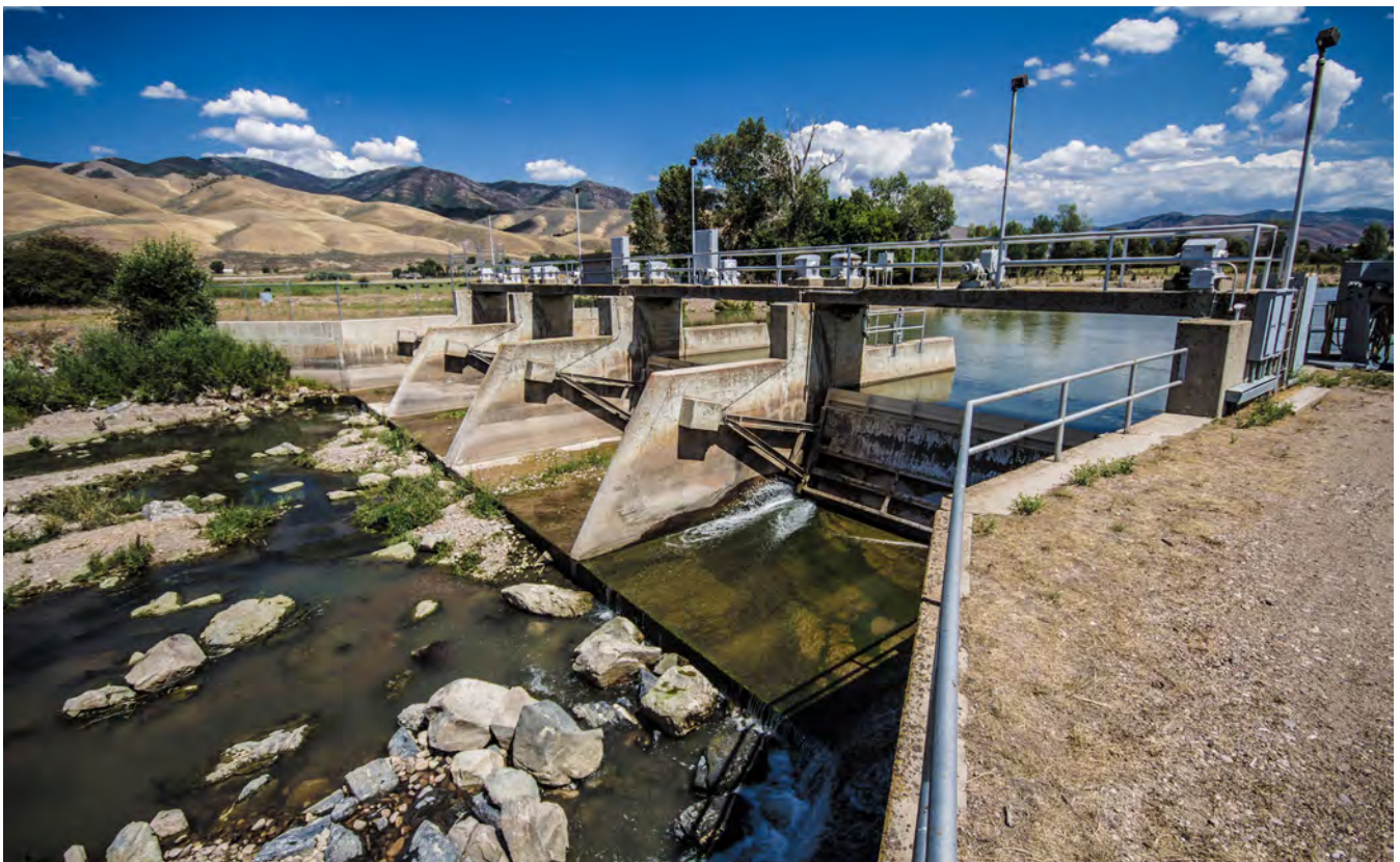
Fig 2.2: Dewatering downstream of the Stoddard Diversion.
